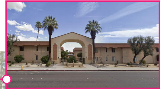
2 STORY APARTMENT COMPLEX
